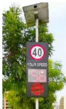
Figure 1. Signaling supply system with photovoltaic panel
